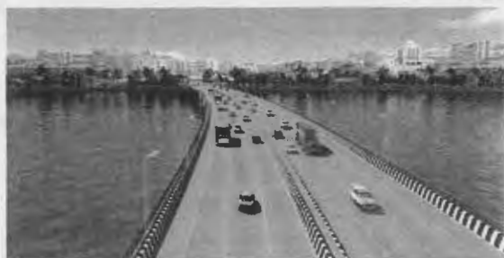
(出典: Mumbai Metropolitan Region Development Authority)
